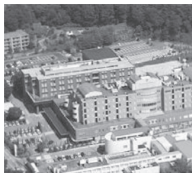
IUHW Hospital (Main Hospital) Number of Beds: 408
